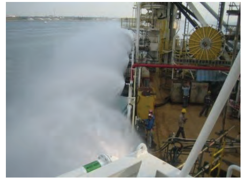
Rig Cooling in Singapore Yard
